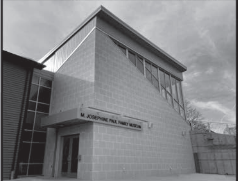
Community Arts Center of Cambria County: Museum Addition Johnstown, PA
